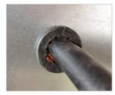
**Step③:** Wrap the cable with the right size cable conduit, and fix the cable conduit to the bulkhead panel passing through the panel hole.
