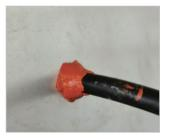
**Step@:** HK-300 type class B15 firestop putty pad is wrapped on the exposed side of cable conduit, to seal the gap between cable and cable conduit, cable conduit and panel.
