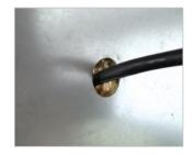
**Step():** Open a fitted hole on class B15 bulkhead panel to install the cable and conduit, according to specifications of cable and cable conduit.
