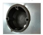
**Step():** Open a fitted hole on class B15 bulkhead panel to install HK-200 type class B15 cavity wall box.
